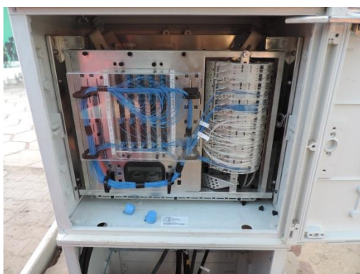
Fig. 13 Level-1 splitter inside the FDT
